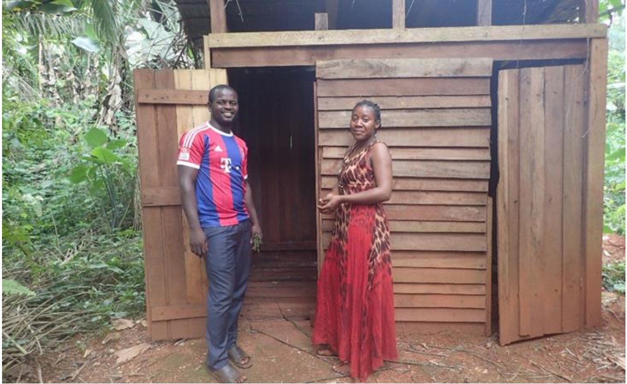
Example of a latrine constructed at household level by community members with technical support from health scouts. Photo Credit: Olivier Njounan, WWF-Cameroon
